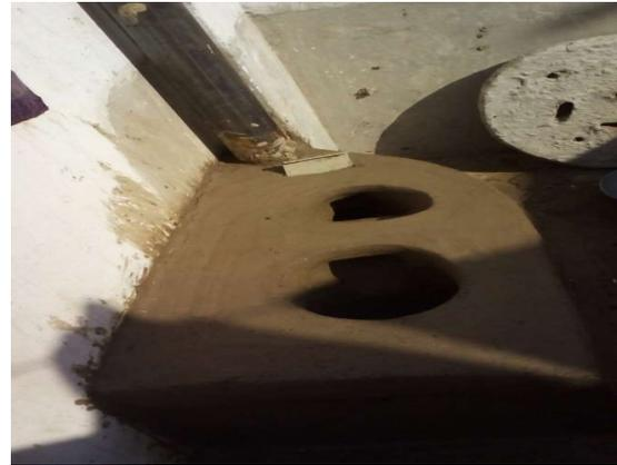
**Fig.3.2 Process of making smokeless chulha by RVIT College, Bijnor**
