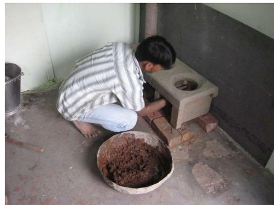
**Fig.3.3 Process of making smokeless chulha by RVIT College, Bijnor**
